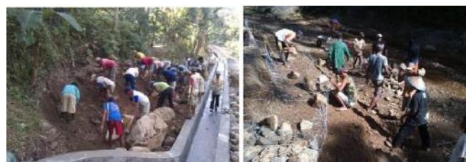
Fig.8: Check dam construction as a project based on community adaptation plans
